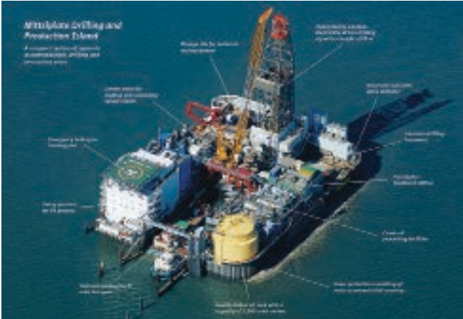
The Mittelplate platform features separate living, drilling and process areas. (Courtesy Wintershall Dea)
