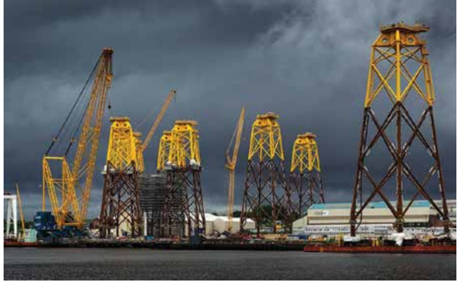
ABOVE: The Wallsend yard is completing assembly of the Moray East wind farm jackets. BELOW: The yard in Senegal is supporting construction of the Greater Tortue Ahmeyim LNG jetty. (Images courtesy Eiffage Métal)
